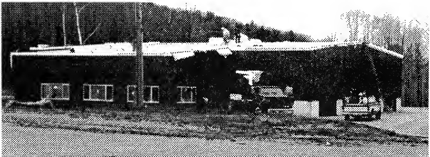
Garage nearing completion of the close in
